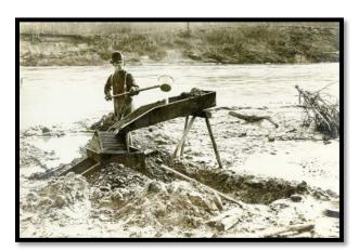
The sluice box and long tom helped the miners process more dirt at a faster rate. Small strips of wood, called riffles, were nailed along the bottoms of these devices to trap the gold as the water washed the dirt through the trough.
