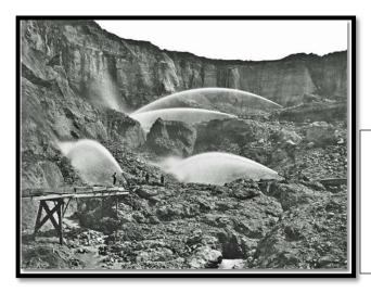
A single water cannon could fill 82 swimming pools in only an hour. The power of a water jet was strong enough to move a school bus.
